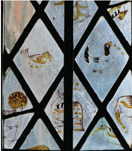
FIG. 17 – Alston Court. Quarries with humorous images of birds in the south hall window.
