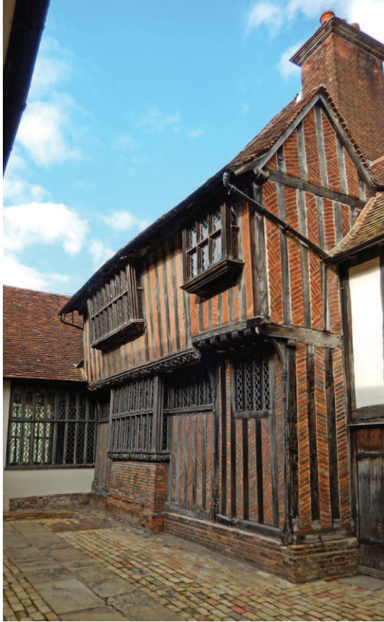
FIG. 16 – Alston Court. The interior courtyard from the south: the hall window is straight ahead and the bay window of the rear parlour is to the left.
